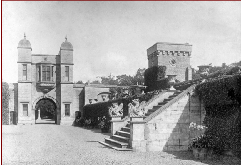
The Gatehouse c1910
